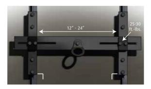
4. Insert Set Screws in bottom two holes of all S-5 Clamps. All Set Screws must face same direction. Ensure all Set Screws will compress against roof seam when fully installed.
